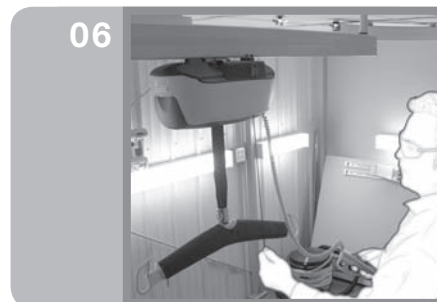
Ceiling lift and charger installation
