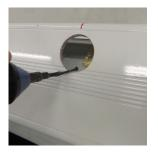
**Step 10**Remove sharp edges on both sides with appropriate tool
